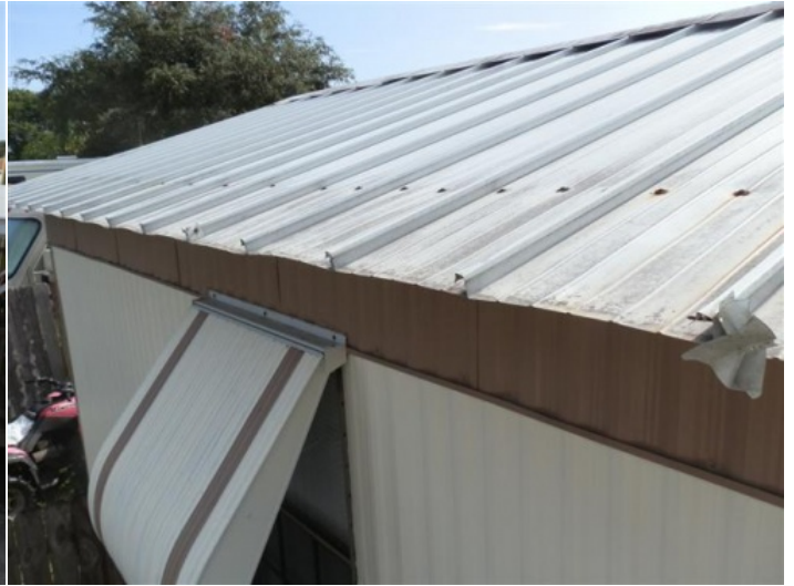
Metal Fascia Has Been Removed
