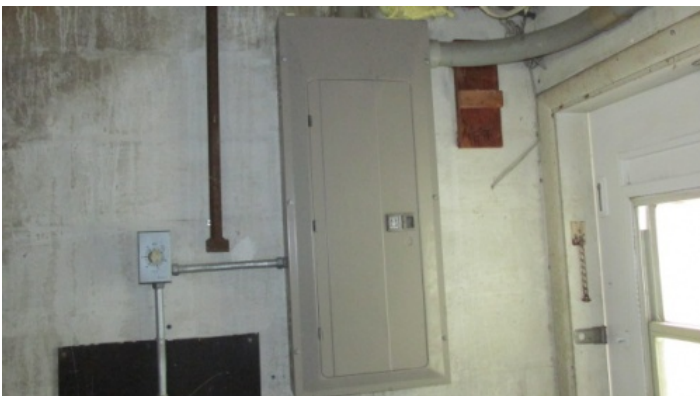
Electrical Distribution Panel (cover on)
