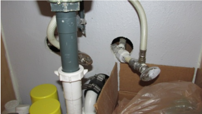
Bath Plumbing (under sink) - shut off valves, flex vinyl water supply lines
