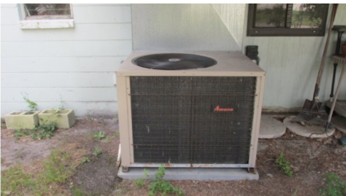
Heating & AC package unit
