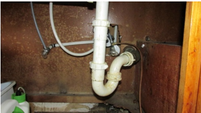
Kitchen Plumbing (under sink) - PEX water supply lines, PVC and galvanized drain
