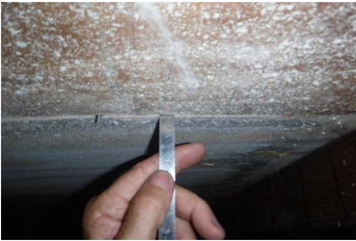
Roof Deck Attachment - 1/2" plywood sheathing
