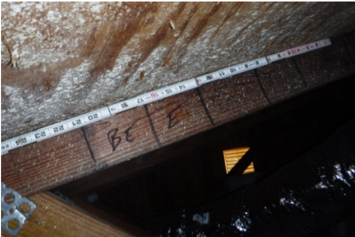
Roof Deck Attachment - 6" spacing on the edge
