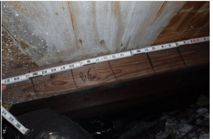
Roof Deck Attachment - 6" spacing in the field
