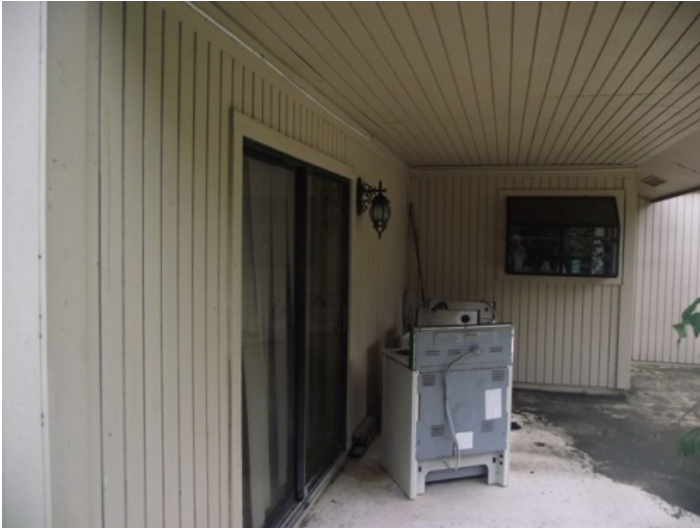
Back Elevation - no openings are protected
