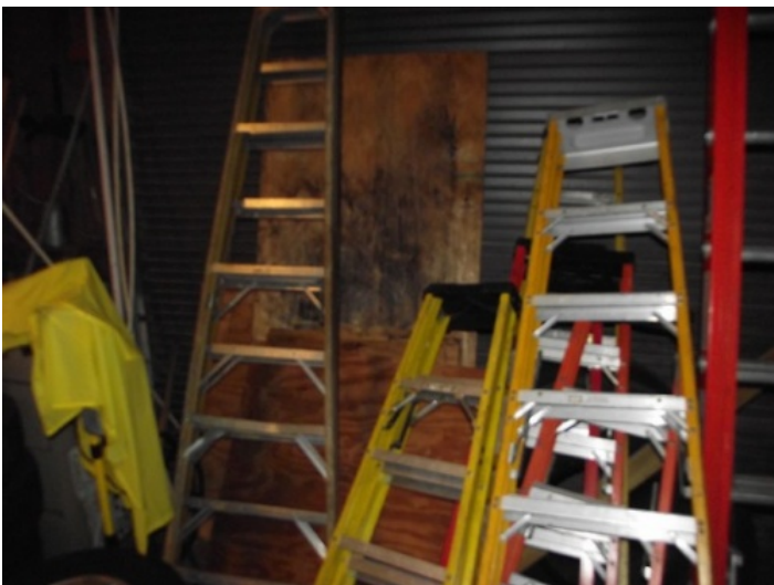
Plywood that does not conform to FBC 2007, no permanent hardware installed
