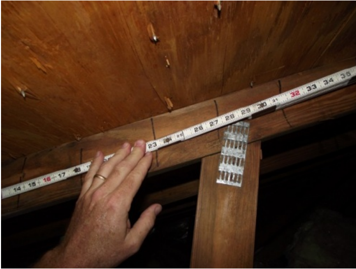
Roof Deck Attachment - 6" spacing on the edge
