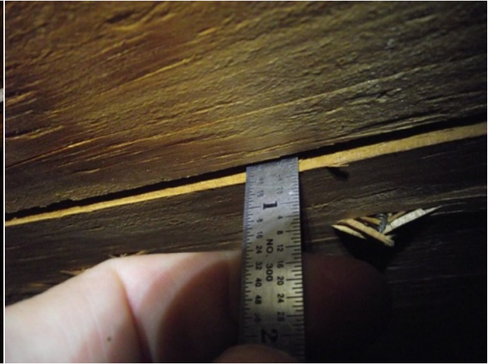
Roof Deck Attachment - 5/8" plywood sheathing
