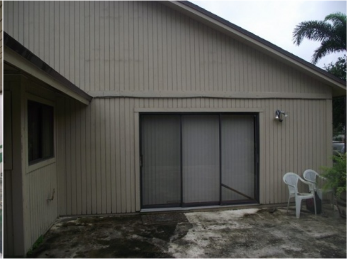
Back Elevation - no openings are protected
