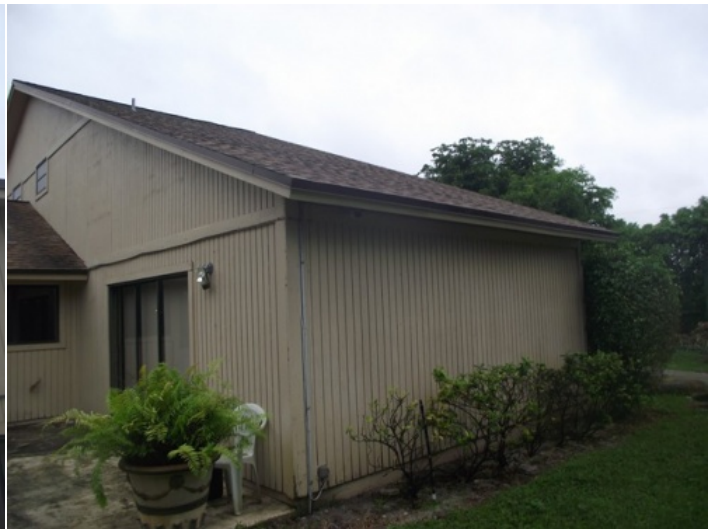
Left Elevation - no openings are protected
