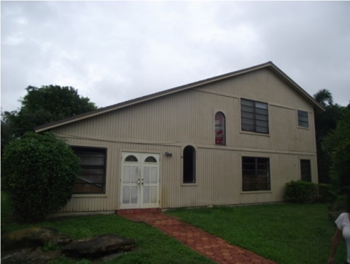
Front Elevation - no openings are protected
