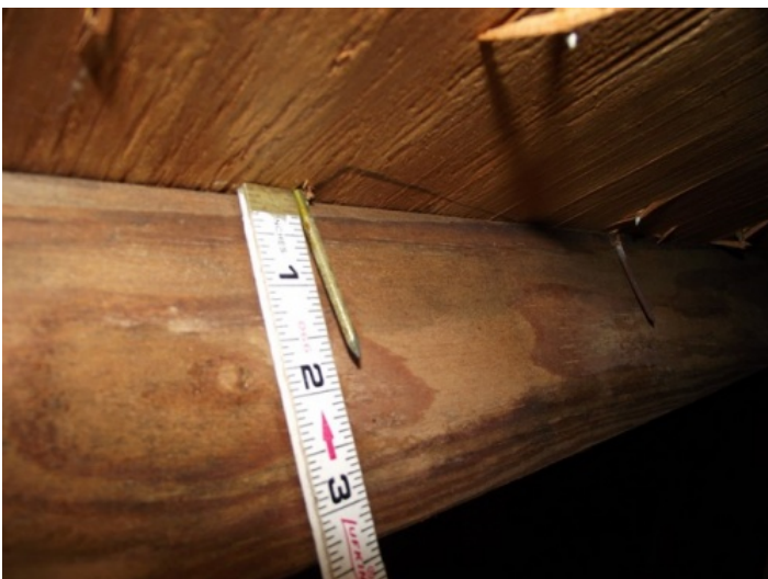
Roof Deck Attachment - 8d nails
