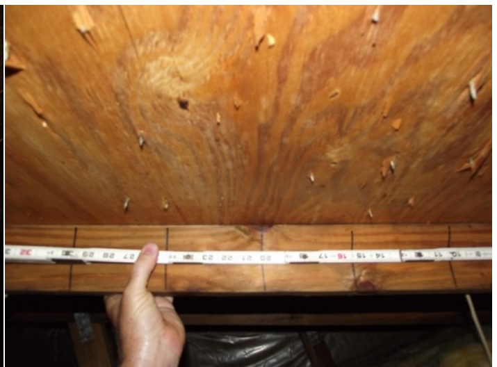
Roof Deck Attachment - 6" spacing in the field
