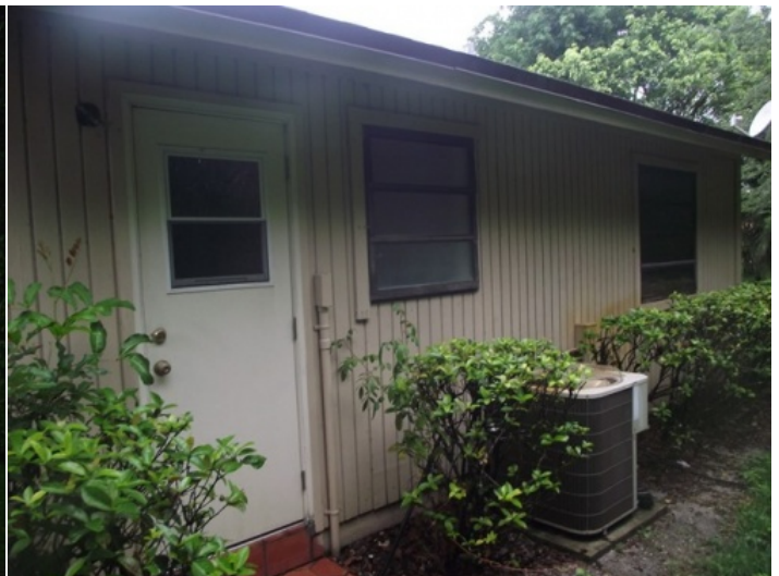
Right Elevation - no openings are protected
