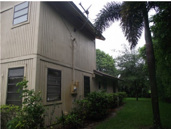
Right Elevation - no openings are protected
