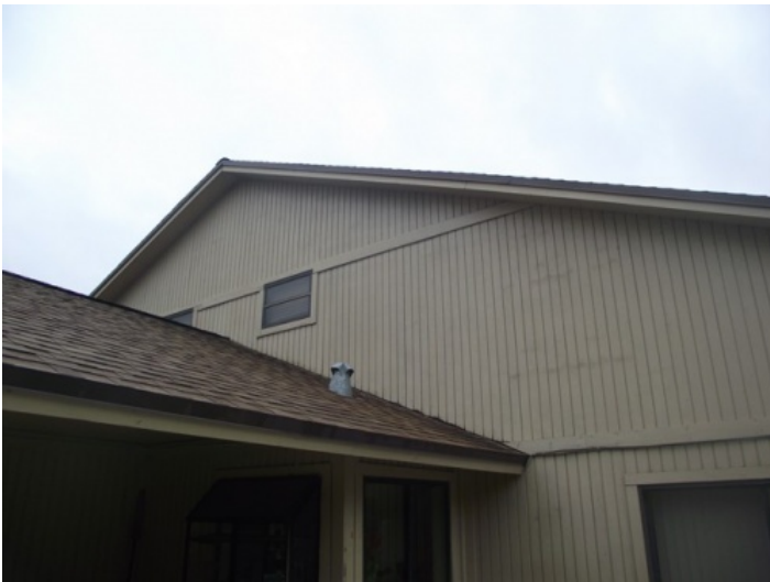
Back Elevation - no openings are protected
