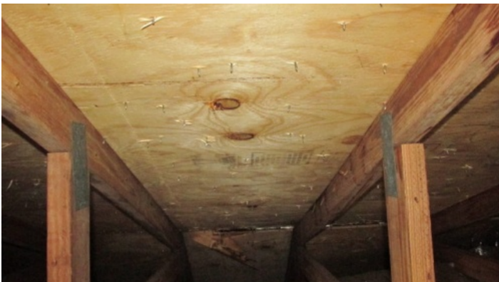
Roof Attic Sheathing - plywood
