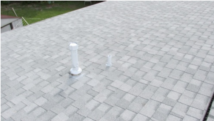
Architectural shingle roof - 2013
